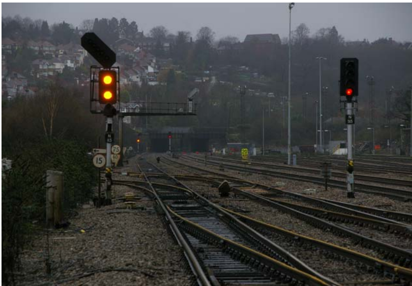
Figure 1 LED Signals at Ebbw Junction, Newport area, 2007 (photo courtesy Andrew Denholm, Network Rail).
